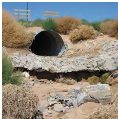
Existing storm pipe drainage onto site
