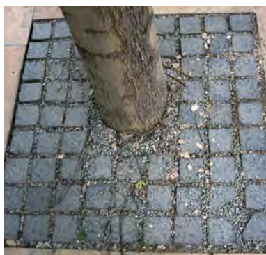
Pervious paving
